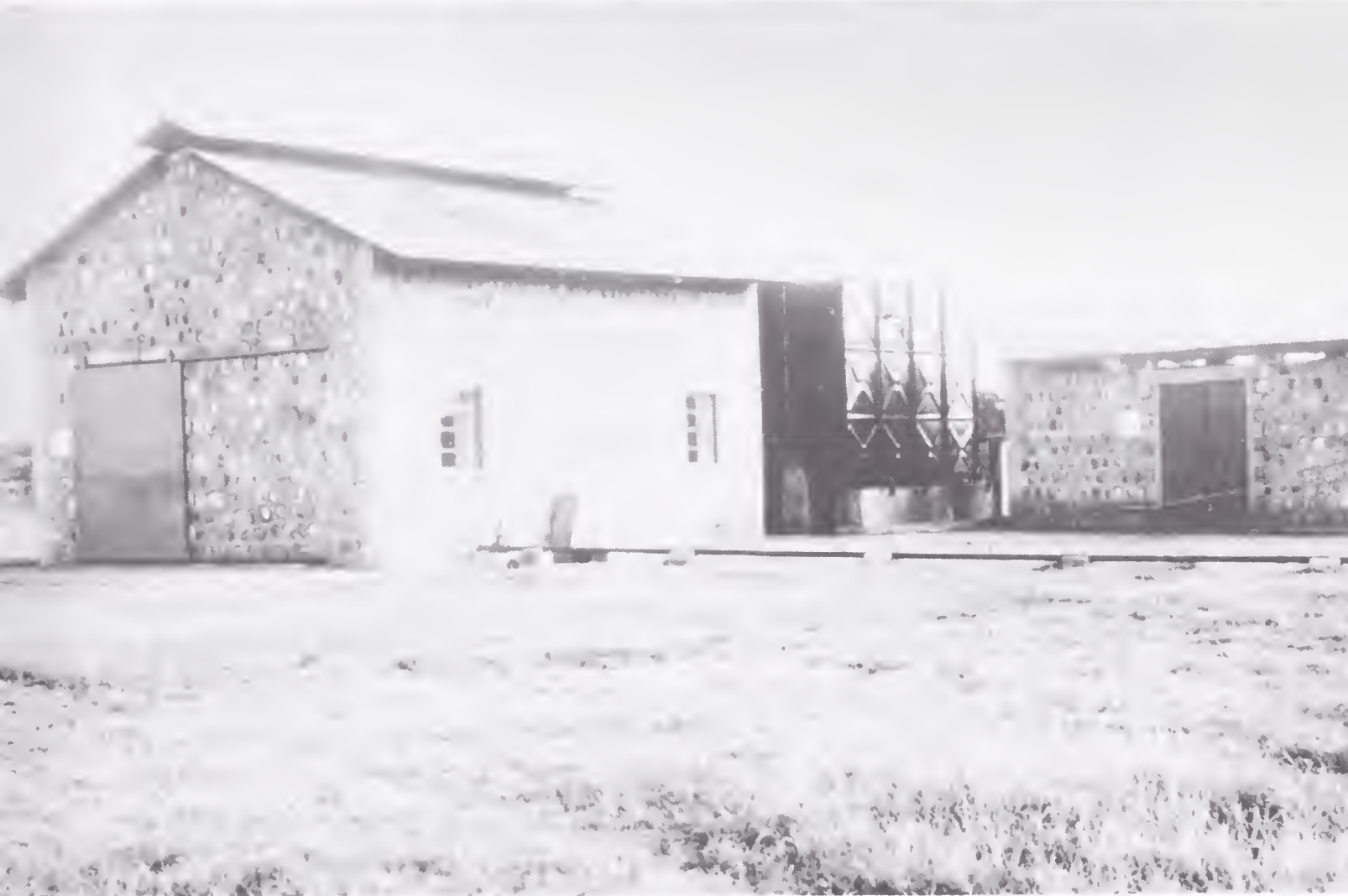
Sennar Dam on the Blue Nile, one of Sudan's oldest dams and major source of electric power for eastern Sudan Courtesy Embassy of the Republic of Sudan, Washington Waterworks at Maridi, west of Juba Courtesy Robert O. Collins
